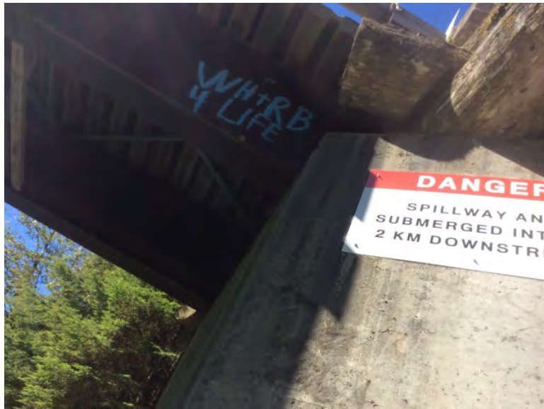
Right Bank Abutment when facing downstream
