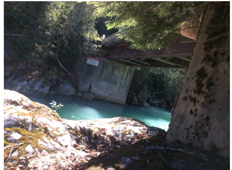
Left Bank Abutment when facing downstream
