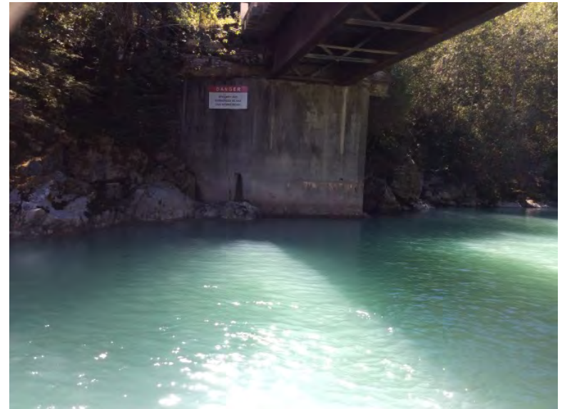
Left Bank Abutment when facing downstream
