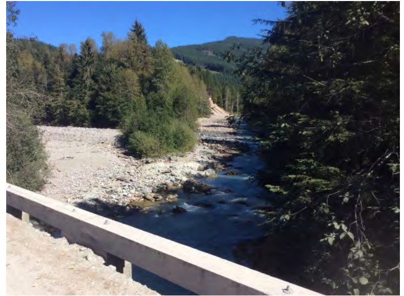
Upstream from Crossing
