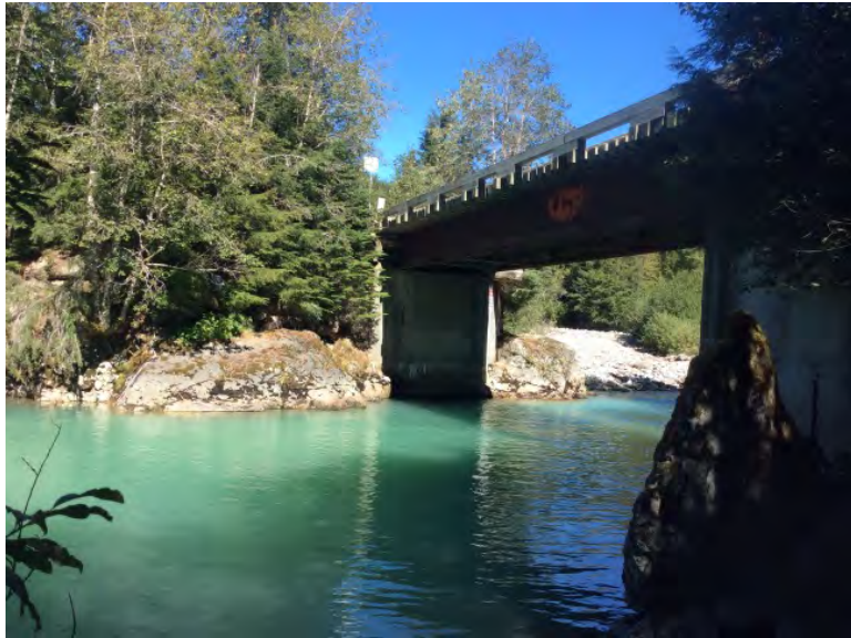
Right Bank Abutment when facing downstream
