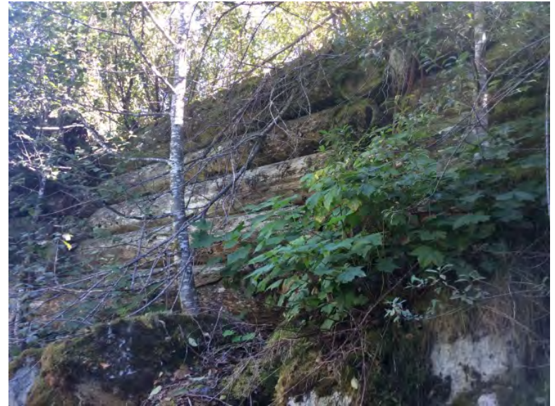
Townside downstream crib wall
