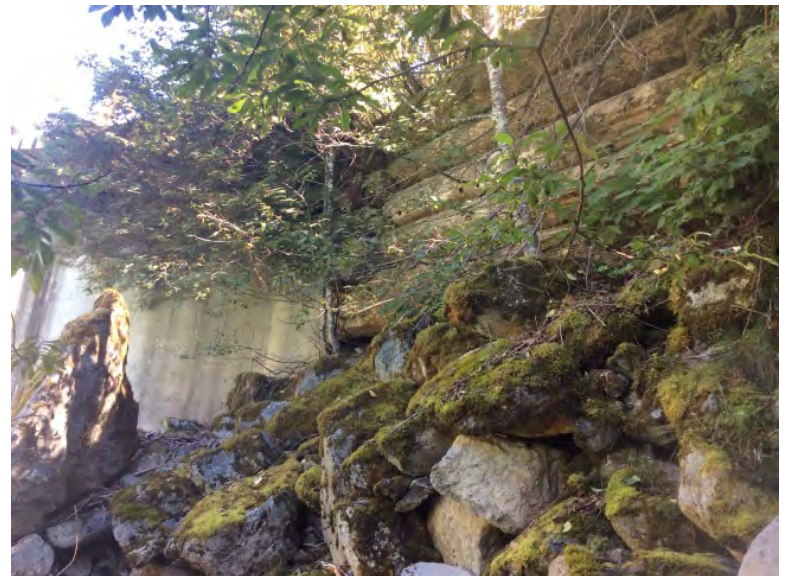
Left Bank Abutment when facing downstream
